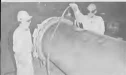
Welders G. Tromp and M. Lopez (r) join two pipe lengths in Welding Shop to make 80 ft. long sections.
